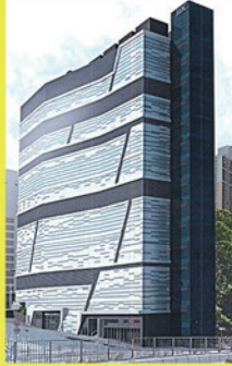
Data Centre - Industrial Building (2020)
