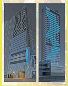
Hotel and Commercial - Heung Yip Road (2019)
