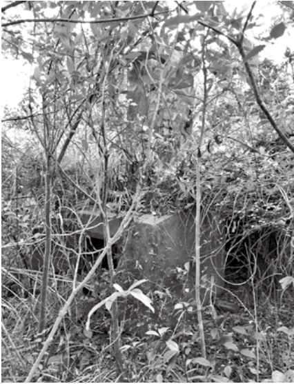
Figure 25: A stove near the water tank
