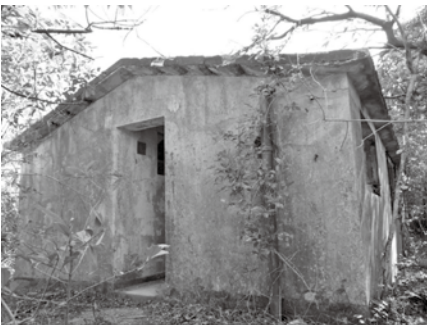
Figure 22: A building near the OP on the 390-meter hill
