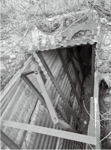
Figure 13: A section of the trench protected by concrete roofing
