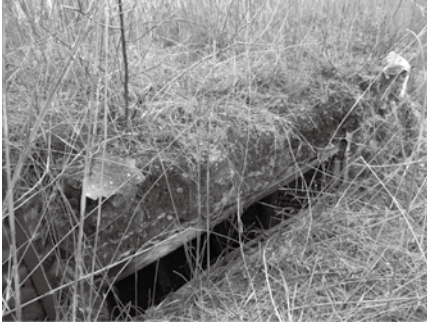
Figure 8: An underground OP near the building
