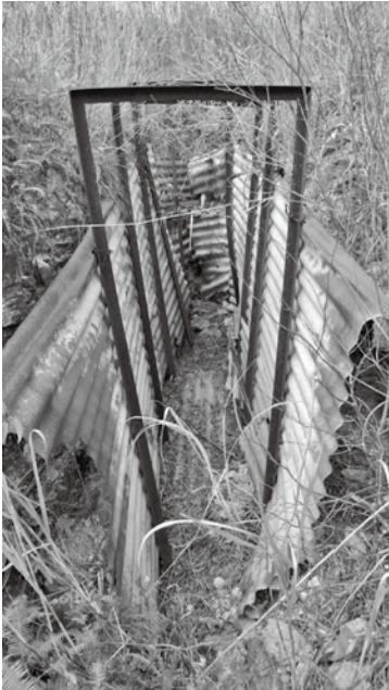
Figure 10: A trench at Wang Lek
