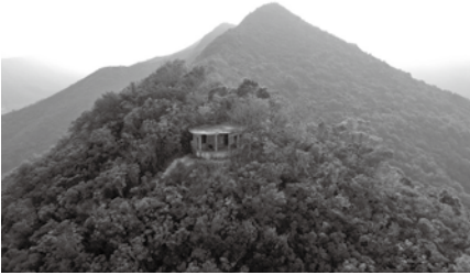
Figure 21: Setting of the OP on the 390-meter hill
