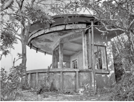
Figure 20: an OP on top of 390-meter hill
