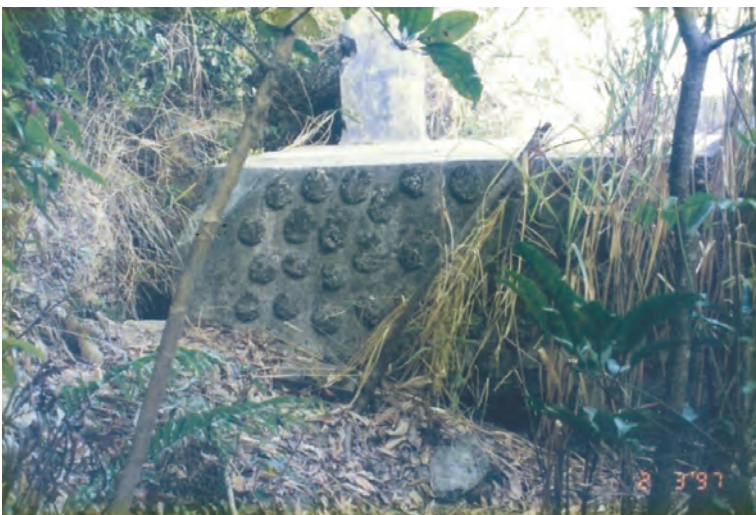
Right side rear, entrance (obscured), airshaft on roof. (March 1997)
