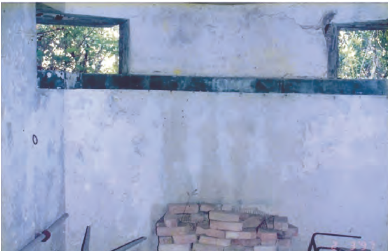
Interior looking forward. (March 1997)
