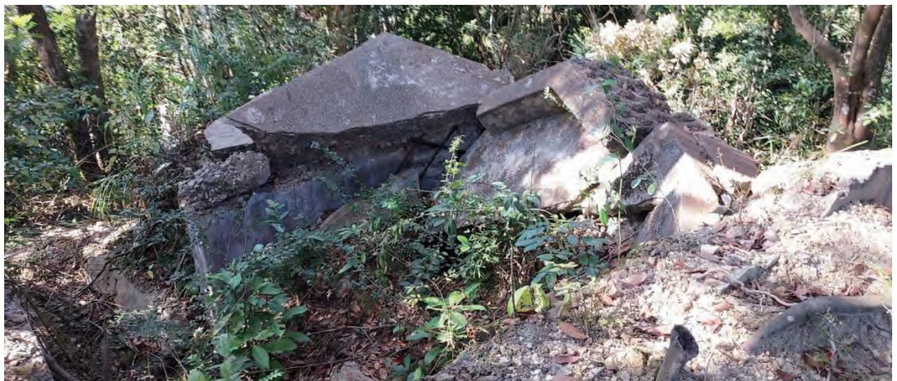
Top view of OP ruins. (4 January 2022 by Lawrence W.C. Lai)
