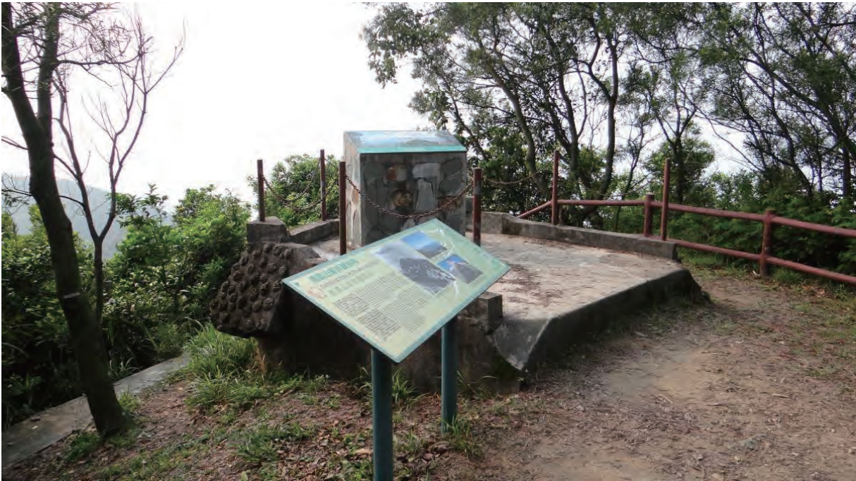
High West OP converted into a public viewing deck with an information board next to it. (April 2016 by Y. K. Tan)
