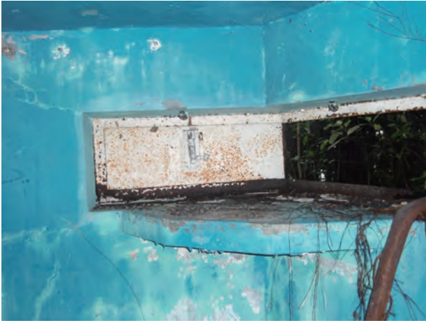
Interior front wall with loophole, one cover missing. (August 2013)
