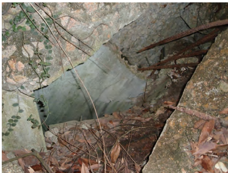
Interior of ruined OP. (December 2009)
