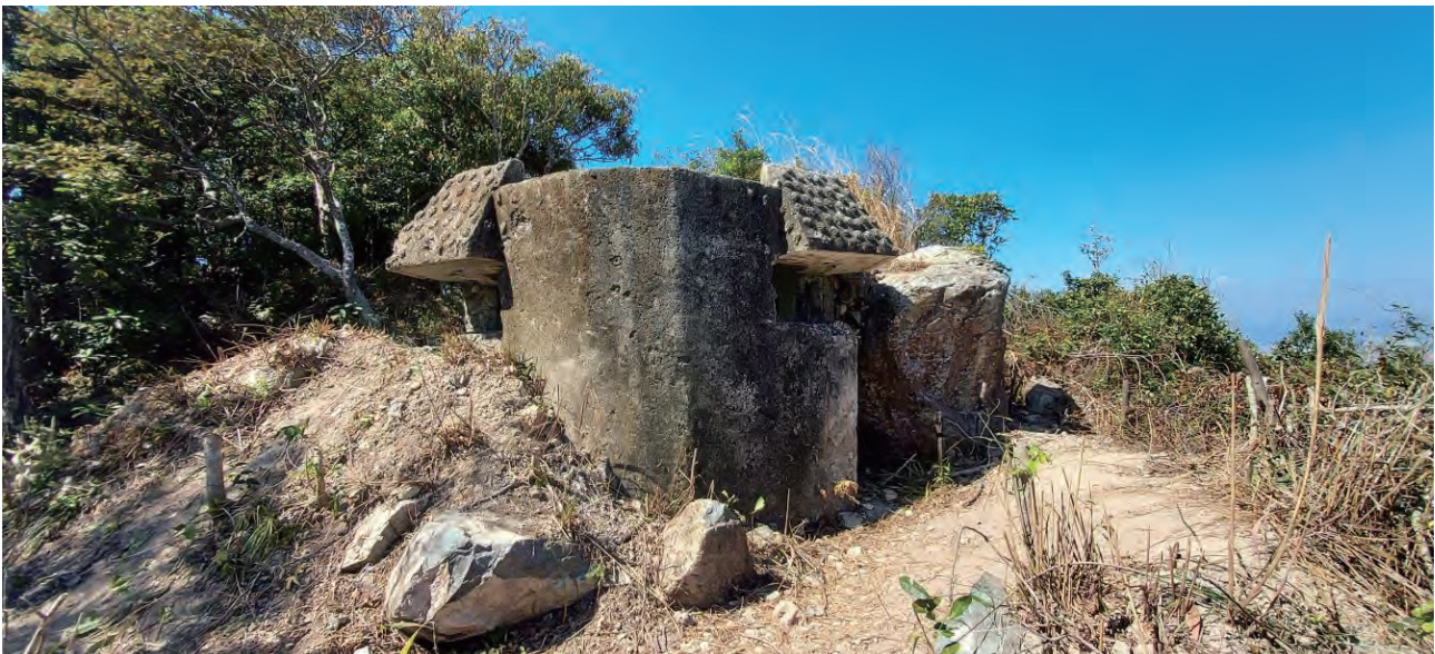
Front view: Lower stone course along the right front found in 1996 (see top left figure at page 48) has gone. (6 February 2021 by Lawrence W.C. Lai)
