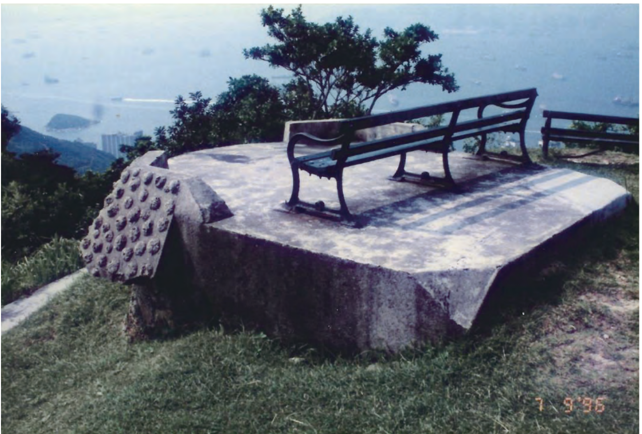
Left side and roof. (September 1996)
