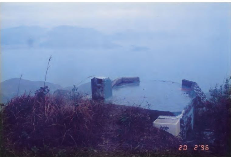
Roof from above and behind. (February 1996)
