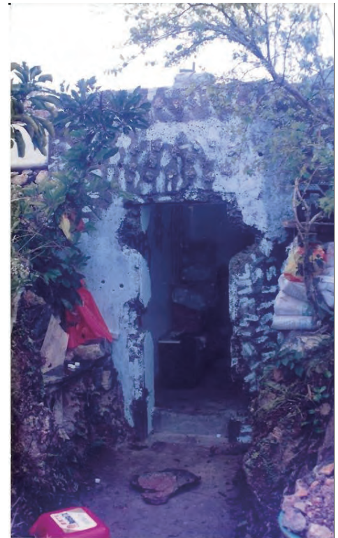
Entrance on right side. (February 1996)
