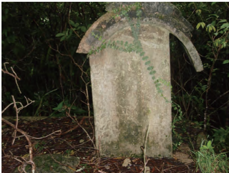
Airshaft on roof. (August 2013)
