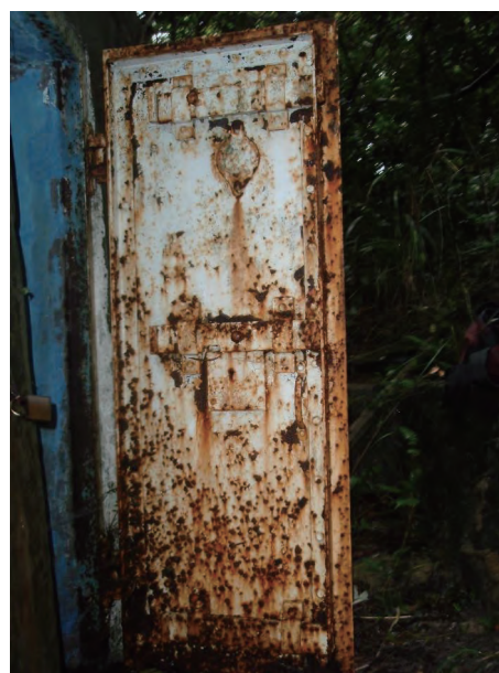
Interior side of entry door. (August 2013)
