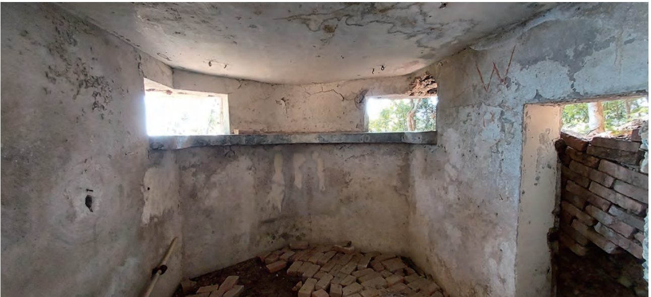
Inside of OP showing its two loopholes and entrance, blocked by bricks and earth. (February 2021 by Lawrence W.C. Lai)
