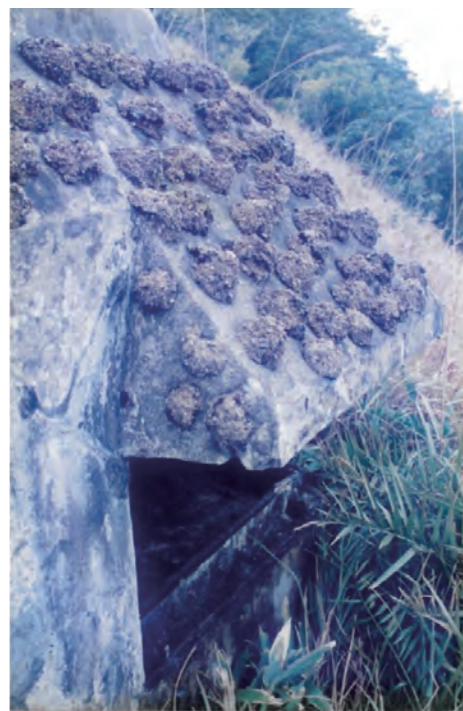
Right front corner. (February 1997)
