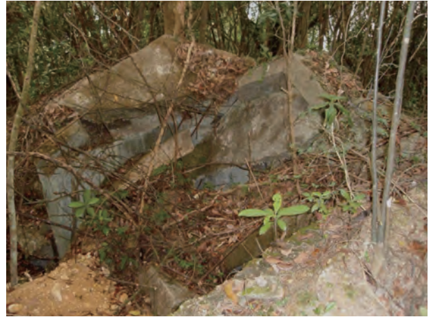
Collapsed roof, entry at bottom left. (December 2009)
