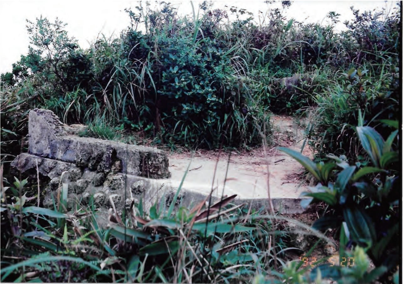
Left side and roof. (May 1992)
