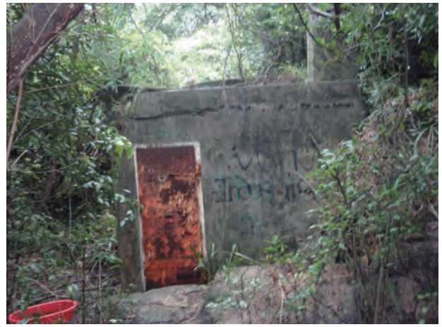
Exterior rear wall and door, airshaft on roof. (August 2013)
