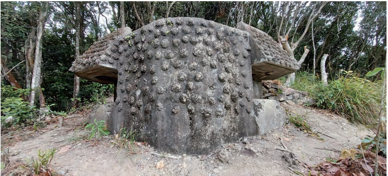
Front view. (31 January 2022 by Lawrence W.C. Lai)
