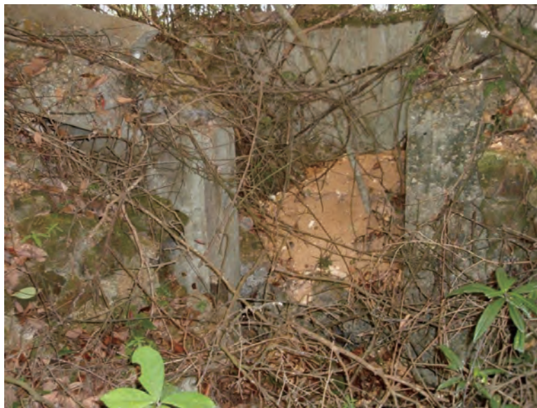
Entry looking in. (December 2009)
