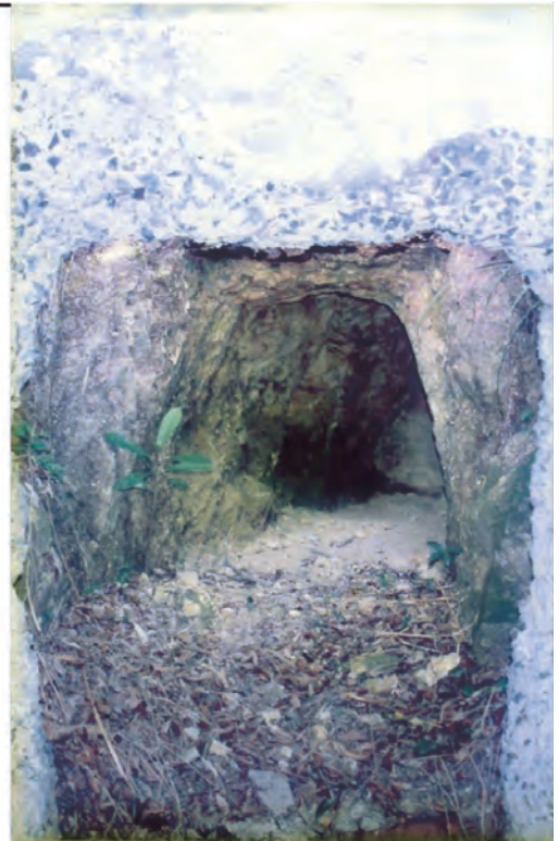
Hole through back wall leading to tunnel entry. (March 1997)
