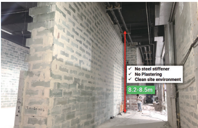
Figure 1: High Wall Erected with GREENTECH Gypsum Block
