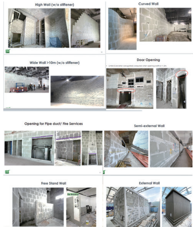
Figures 7 & 8: Applying GREENTECH Gypsum Block to Different Building Functions
