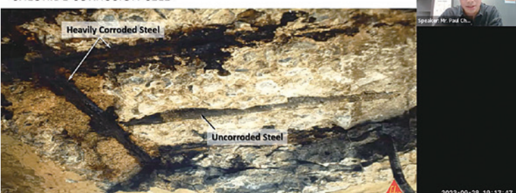
CHLORIDE CORROSION CELL
