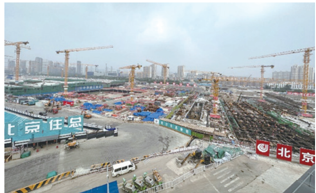
Beijing Sub-Center Railway Station Development
