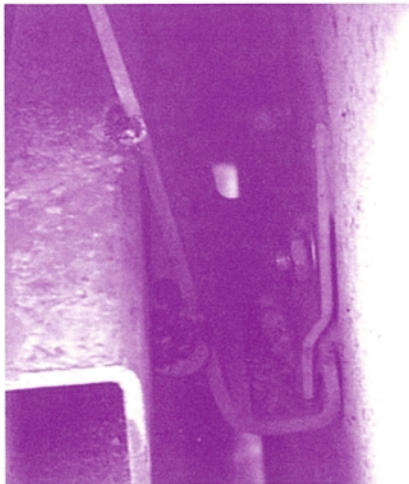
Fig.1 An example of inaccurate fixing.
